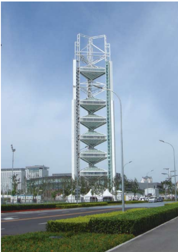
Multi-media broadcasting tower in the Olympic Green
